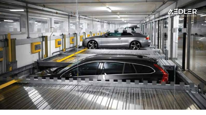
Semi-Automated systems make use of mechanical lift technology with the addition of electricals and PLCs to make the car platform move. The system works to store cars from 2 levels high up to a maximum of 6 levels. All parking places can be selected and used independently. The column-free construction ensures that vertical supports are only required at every 2 or 3 parking spaces next to each other.
